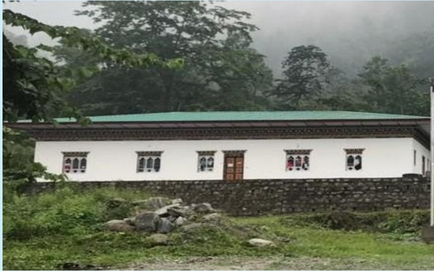
Figure 2: Community hall turned COVID-19 isolation ward in Minjiwoong
